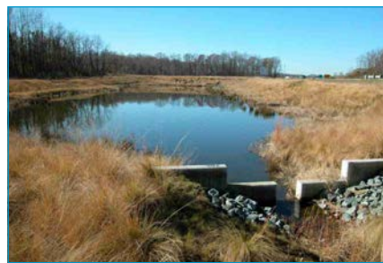
FIGURE 1.2 A large stormwater detention facility. Source: Delaware DOT
