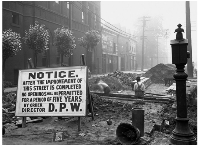
Figure 4.1 Dig-once was deliberate policy of the City in the early 20th century. When a street was opened, re-openings were prohibited for a period of five years to minimize disturbances and to encourage project alignment between utilities and private property owners. Photo from N. Highland Avenue, East Liberty, 1922, Pittsburgh City Photographer Collection.
