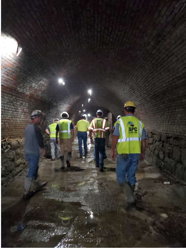
July 2021 Before: Brick structure with major structural defects and wall missing
