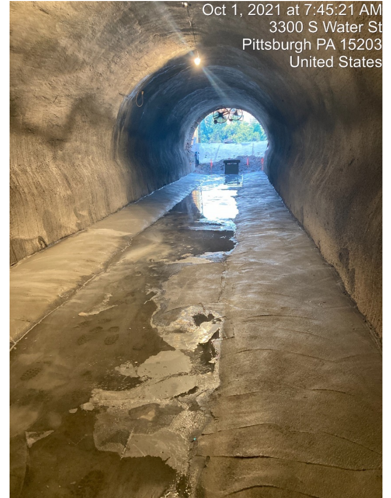
October 2021 After: Full structural lining and new invert
