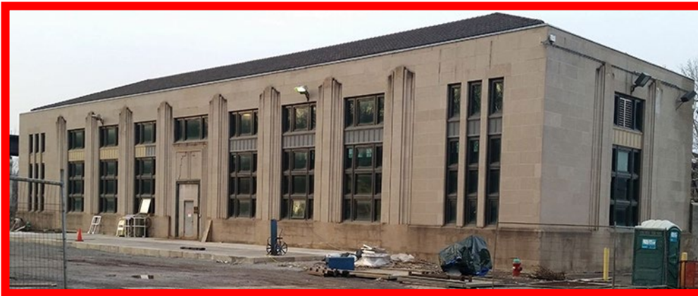
Bruecken Pump Station
