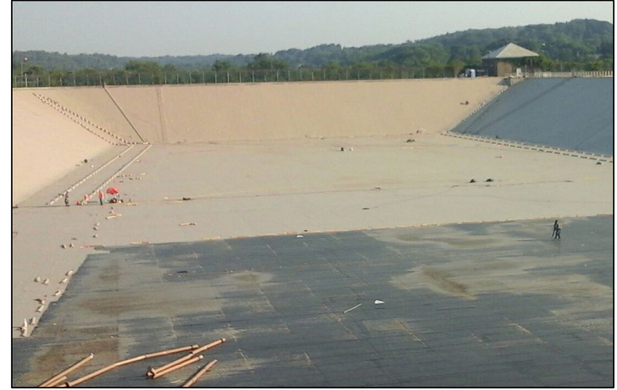
Lanpher Reservoir (Completed)
