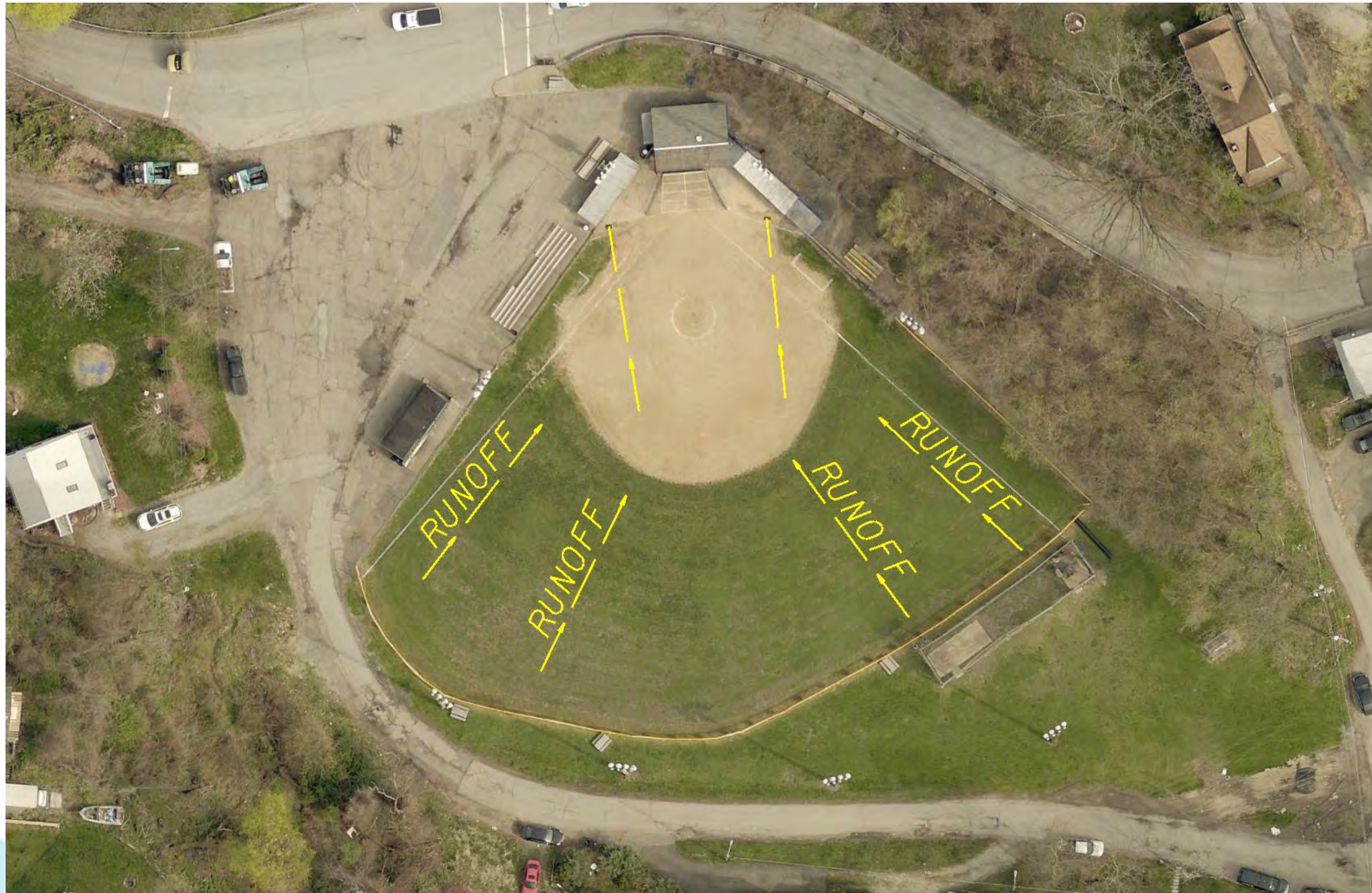
Existing Drainage at VF #2
